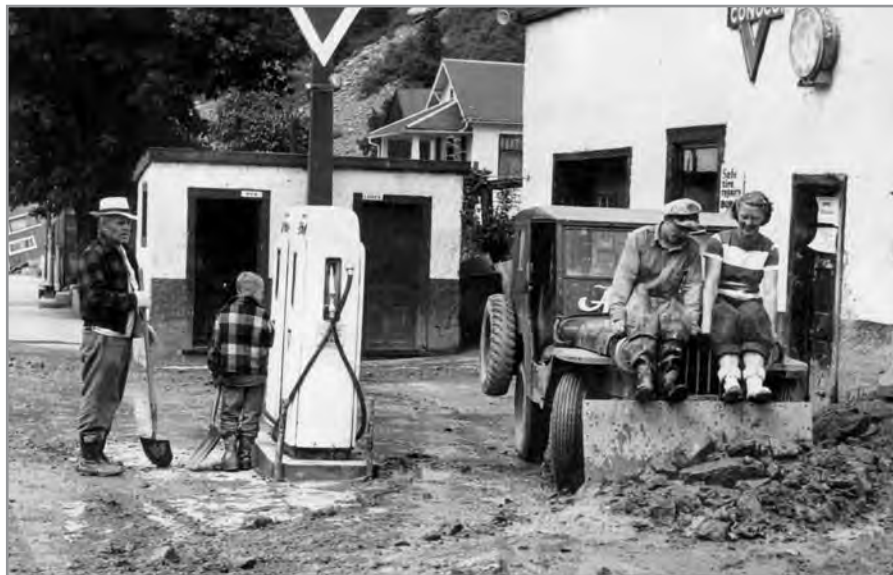
► Joan Fedel and Jack Felin, seated on the hood of a truck, in front of Al Fedel's Conoco Garage on Main Street in Ouray during the flood of 1951.
