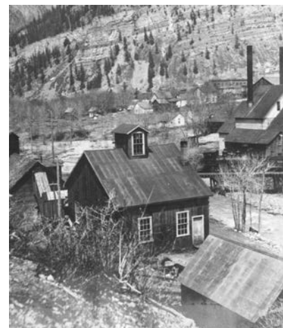
Ouray Power House c. 1905
