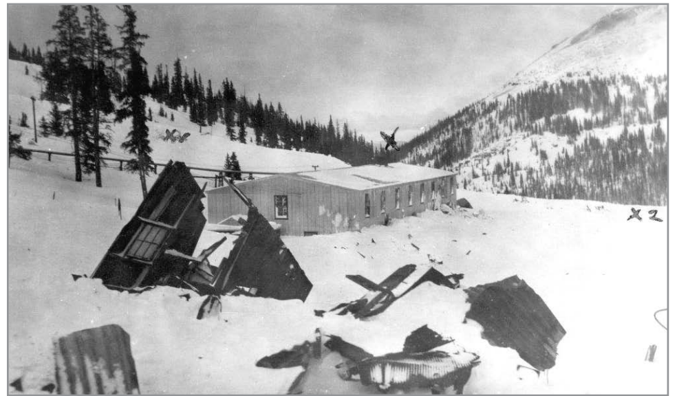
▲ Bottom story of boarding house completely buried by snow slide.
