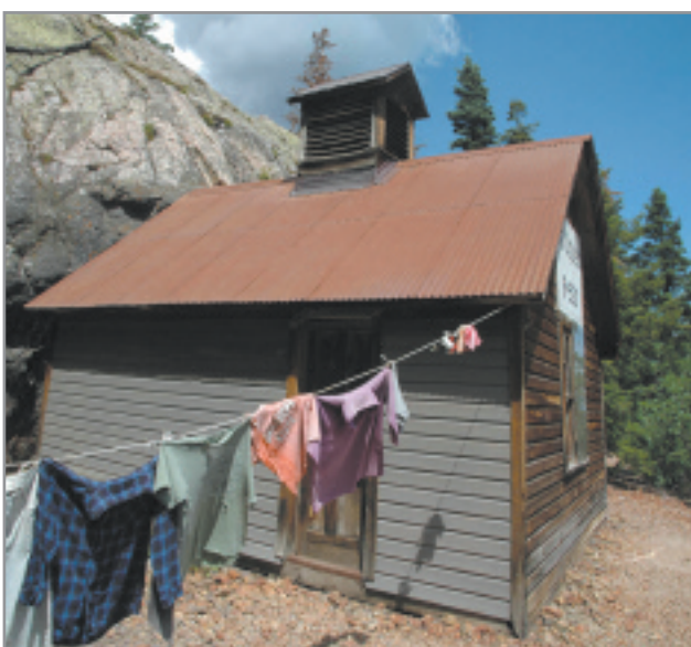
▲ The Neosaha Mine Blacksmith Shop before (above) and after repair.
